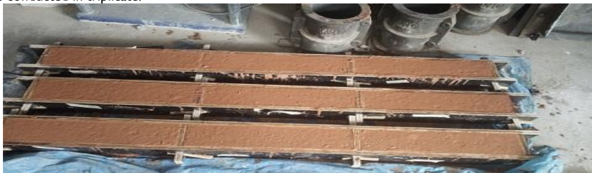
Plate 1: Casting of the reinforced Metakaolin-based geopolymer concrete beams
