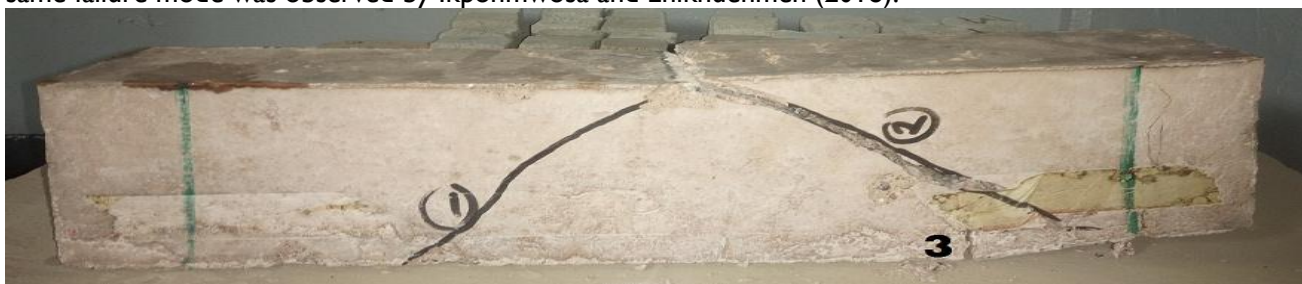
Plate 3: Sample of the failure configuration of the geopolymer beam
