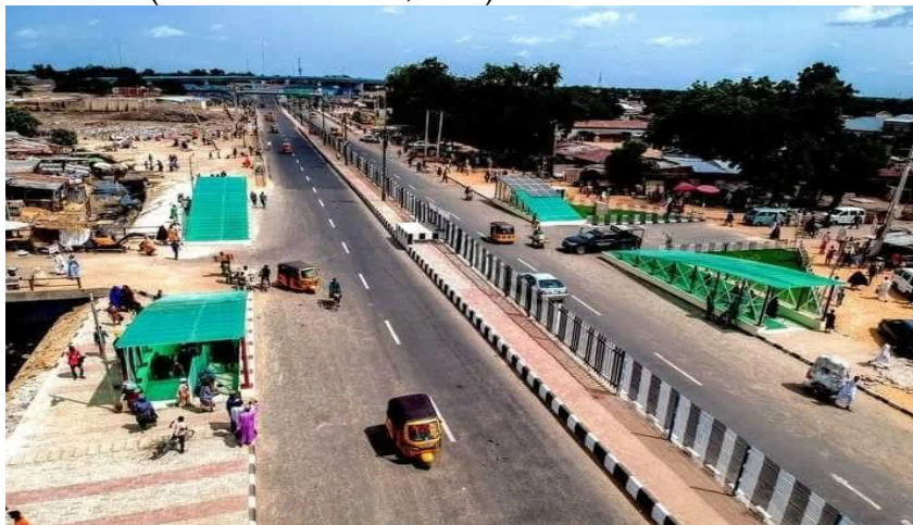
Plate 3: Pedestrian underpass at Gamboru market, Maiduguri
