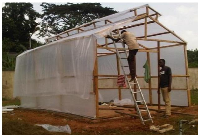
Figure 2: Greenhouse Covering the greenhouse
